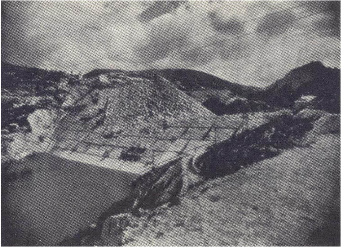
Paradela Dam Concrete Face; 110 m Height; Year: 1956-1958
