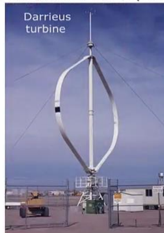
Vertical axis wind turbine (VAWT)
