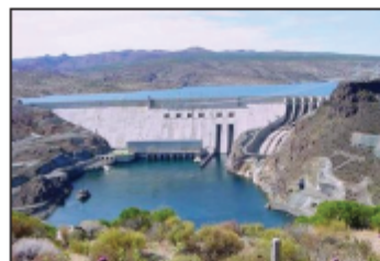
(a) General view of the Piedra del Aguila dam.
