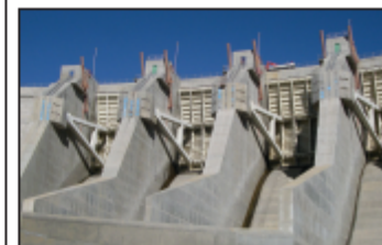
(b) View of the spillway and floodgates.
