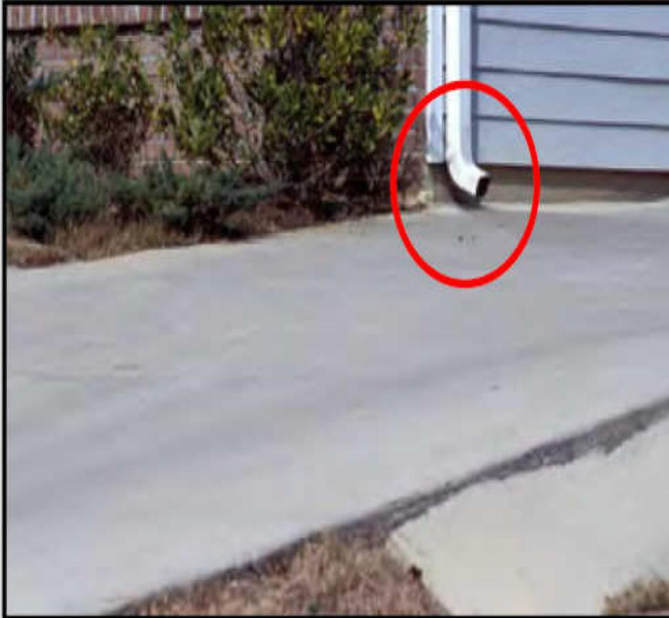
*A directly connected roof drain*
