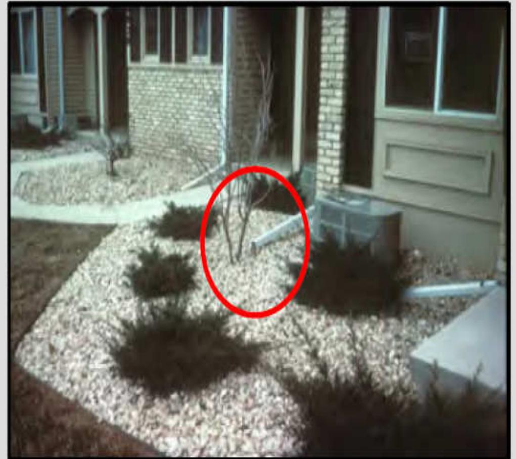
*A disconnected roof drain (drains to pervious area)*
